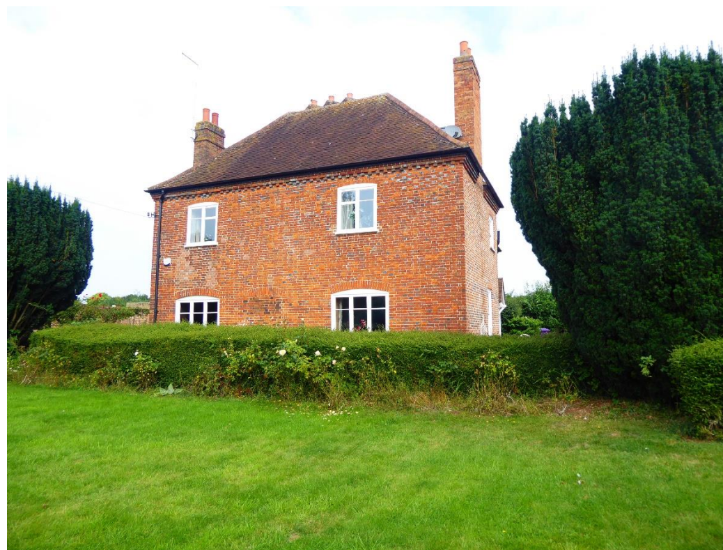
Figure 18: The rear of the Grade II Listed Chesfield Manor Farmhouse
