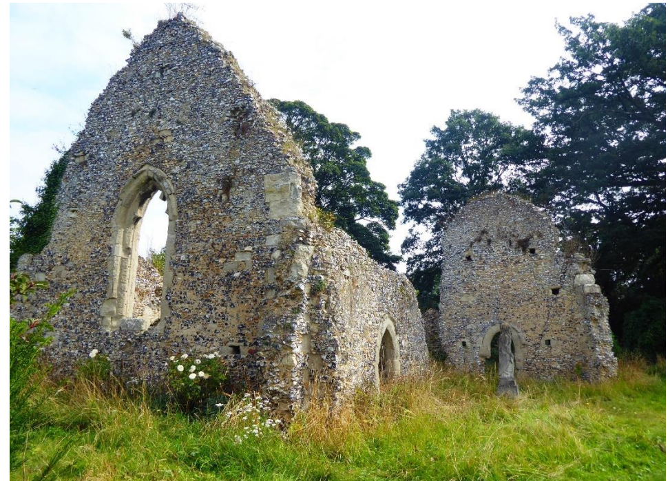
Figure 17: The ruins of Grade II* Listed and Scheduled St Etheldreda Church
