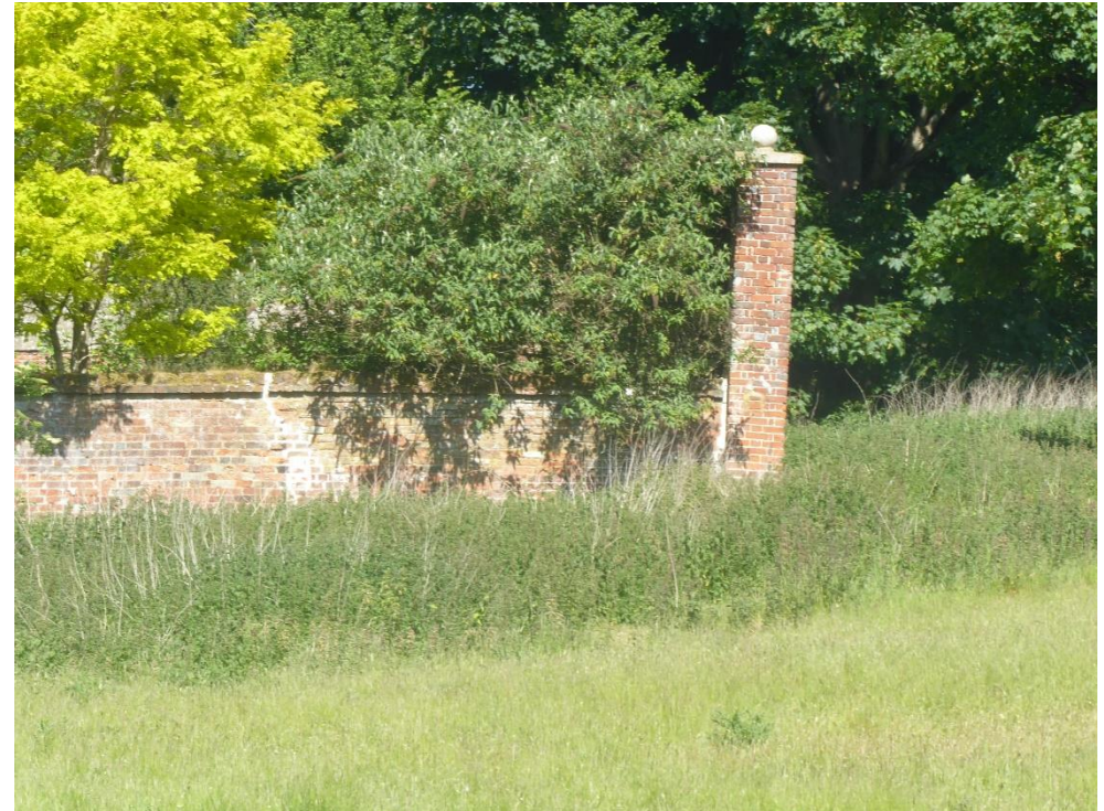
Figure 33: Garden boundary wall surrounding Chesfield Park House
