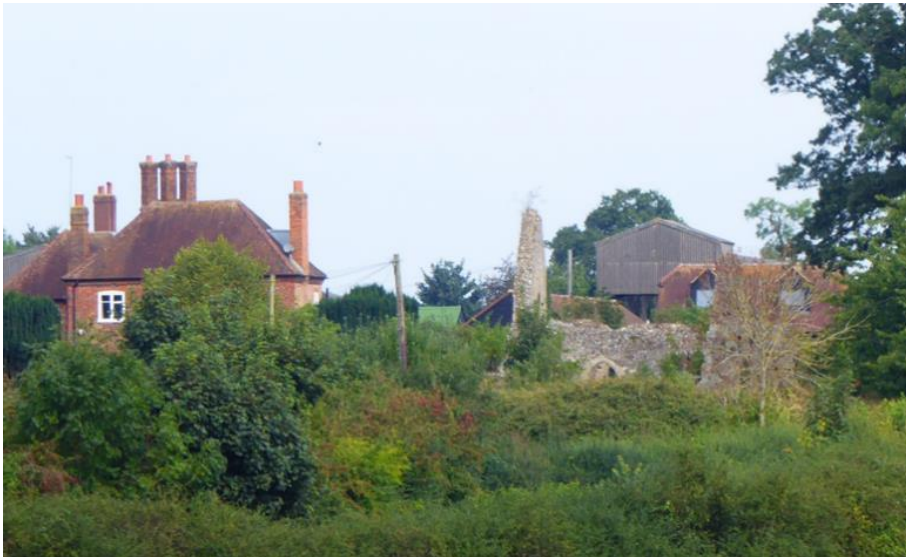
Figure 28: Modern buildings behind Chesfield Manor with corrugated cladding
